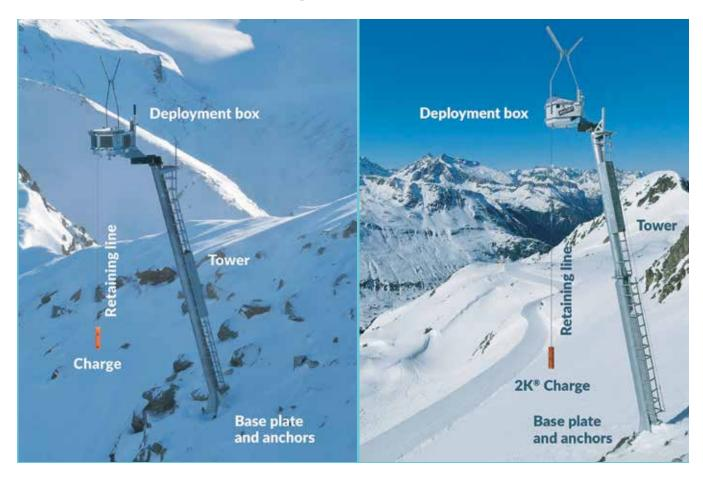
**Project Description:** Installment of "Remote Avalanche Control Systems" (RACS) capable of remote triggering avalanche paths that impact infrastructure and main ski area operations.
